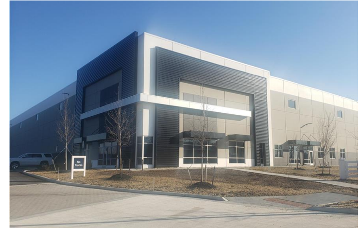
TriMas Packaging New Albany, Ohio, Facility Progress
