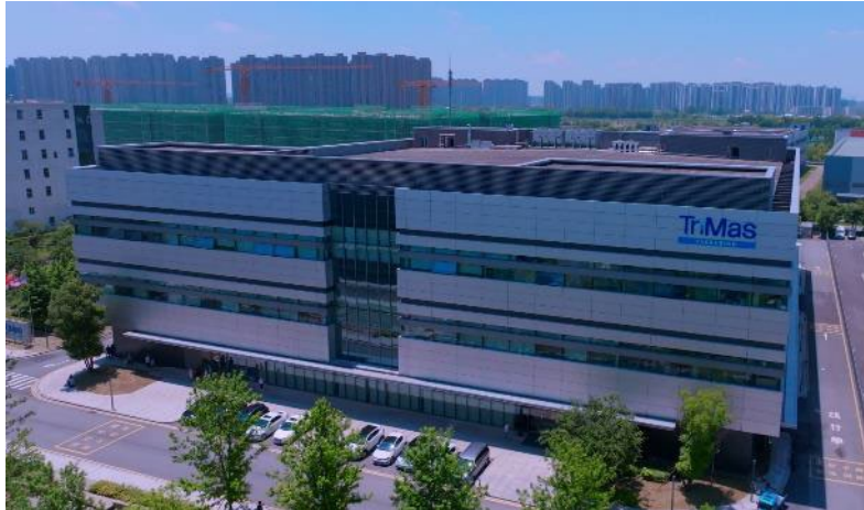
New state-of-the-art facility in Haining, China
